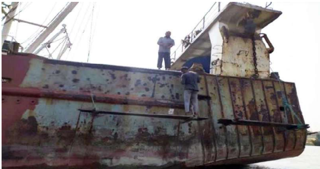
Figure 3: Removing paint from ship (Courtesy: Eva shill)
